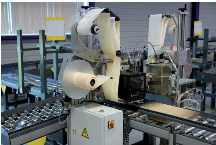
Labeling machine controlled by a L series PLC
